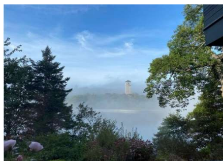
Dingle Tower, Sir Sandford Fleming Park
